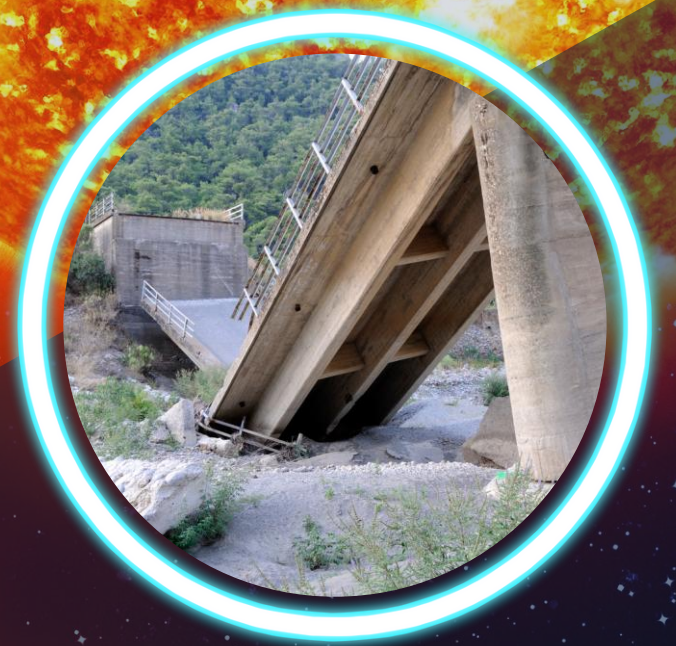
Transportation Cut Off from Earth Quake
